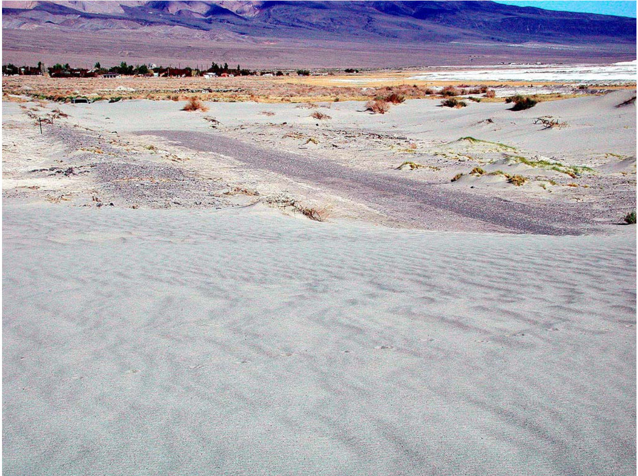
Figure 7.4 – Sand dune that formed across the old State Highway to Death Valley (view looking southeast toward Keeler)
